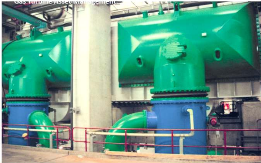
Filter type PR-BW 800 in a power station
